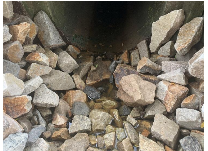
64 Gundalow - 2 (Drainage Course)
