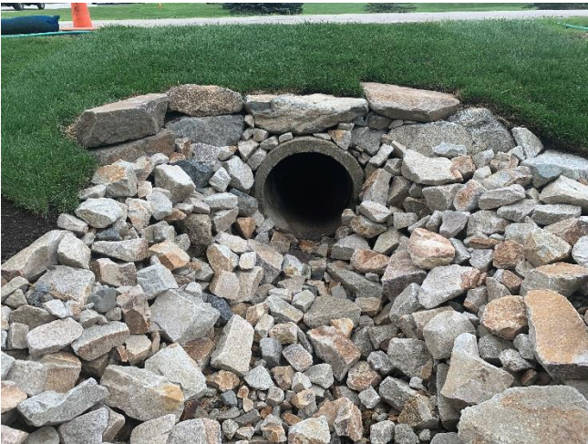
64 Gundalow - 1 (Drainage Course)
