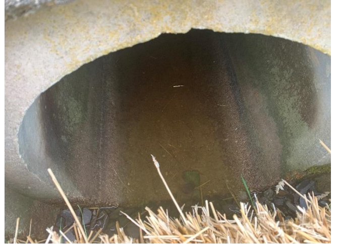
29 Gundalow - 1 (Drainage Area)
