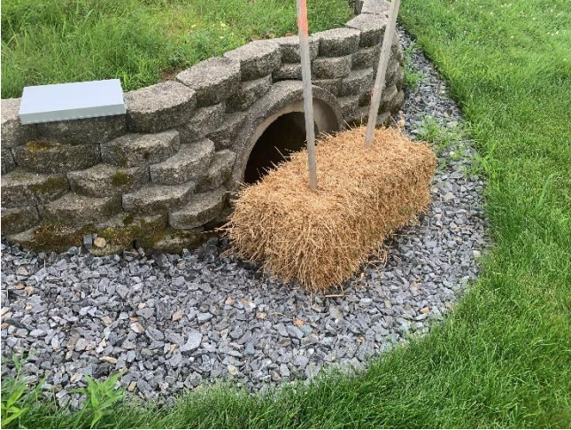
29 Gundalow - 1 (Drainage Area)
